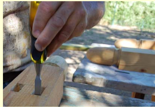
Bobby Wilson chisels one of the many mortises on one of seven posts. © HSFF 2012
