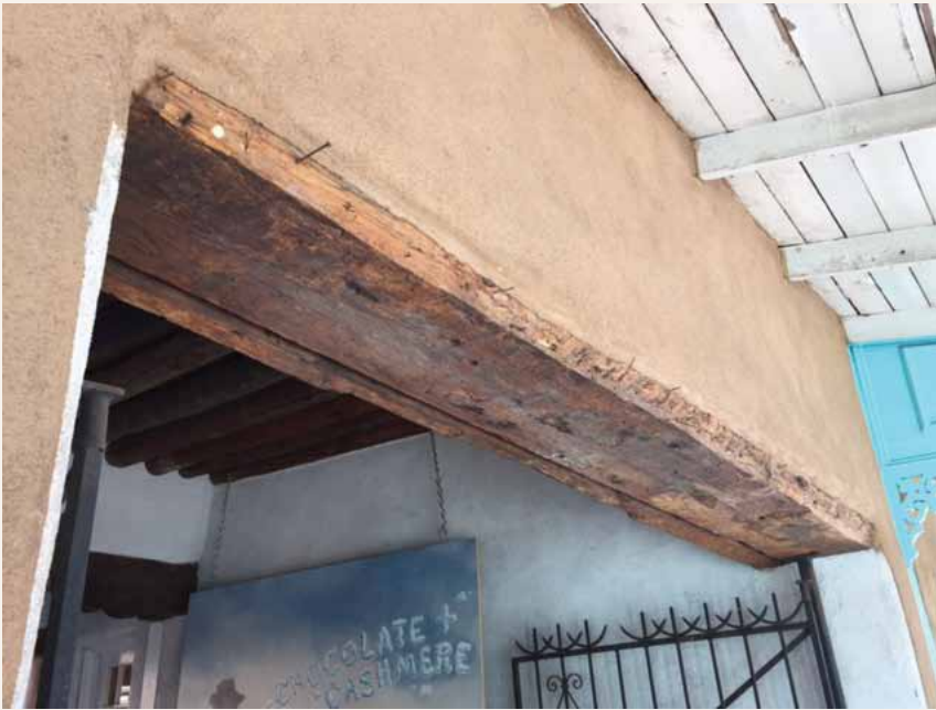
Figure 4. The massive lintel over the courtyard entrance to the Trujillo Plaza was formed from a large ponderosa pine tree that was cut in the early 1690s, around the time of Vargas's reconquest. Note the small tan plug in the upper left corner covering the hole left by one of the two cores.
