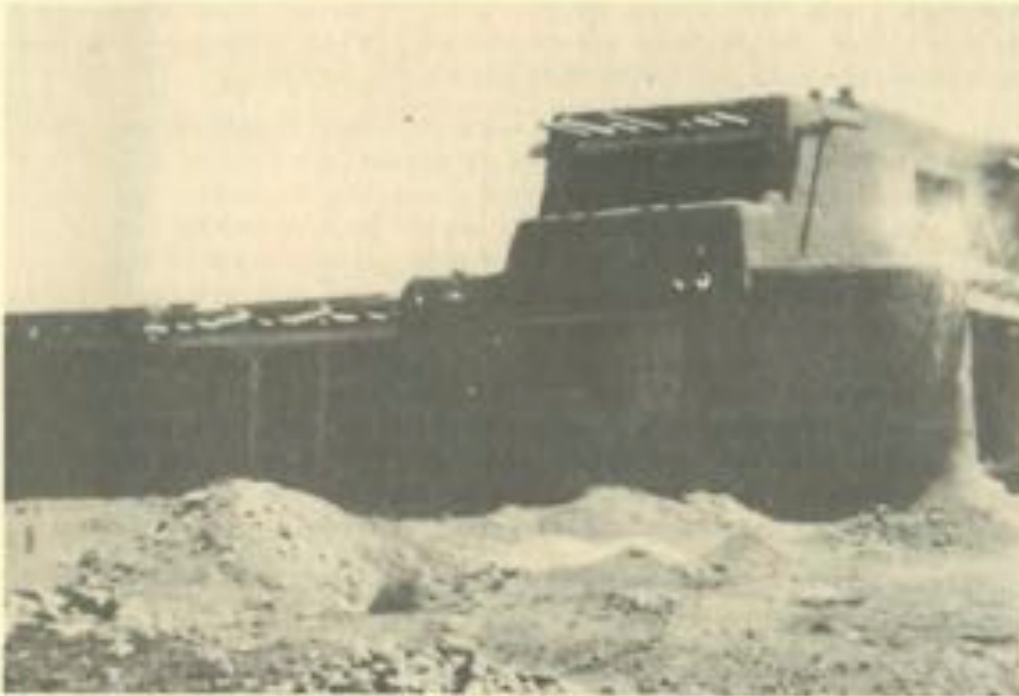
West side of the Carlos Vierra House during construction. Nancy Quintana Collection, State Records Center and Archives, Santa Fe, New Mexico.
