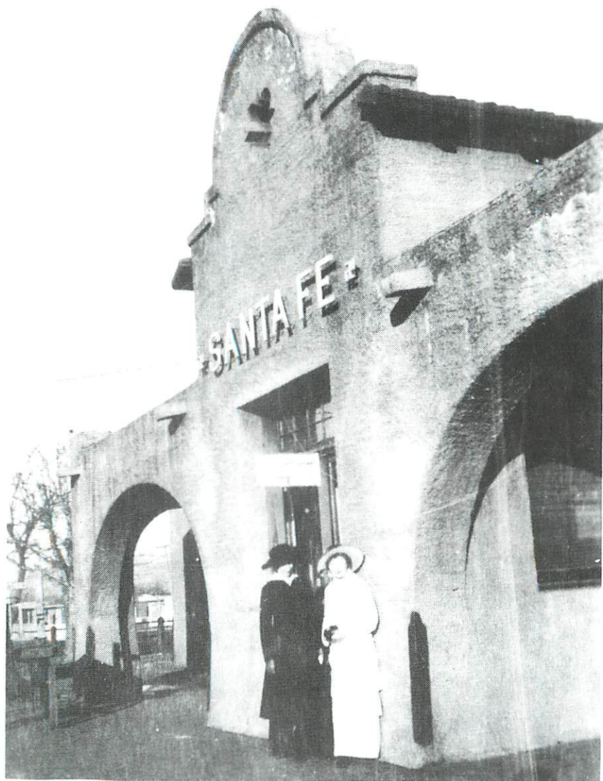
Atchison, Topeka and Santa Fe passenger depot at Santa Fe.
