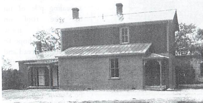
Irvine House view from east. © 1986 Photo by Corinne Sze
