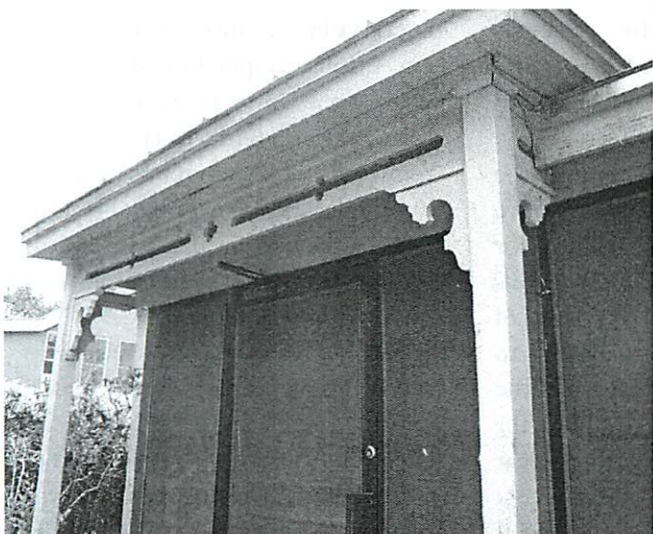
A porch on the back addition, built before 1902, also has decorative wooden brackets. © 2002 HSFF
