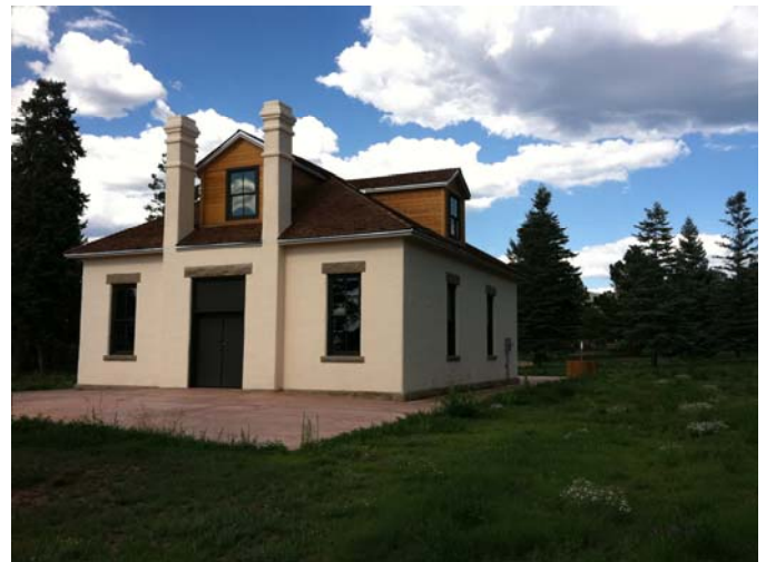
The restored Hydro Electric Plant (above) is the future home of the Santa Fe Water History Museum. Visit it and enjoy the park facility at the northeast corner of upper Canyon Road and Camino Cabra. Photo © HSFF
