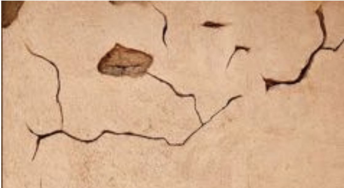
Abstract art? No, wall prep to remud with adobe.
