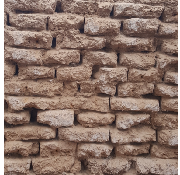
El Zaguán wall during renovations exposing the adobe bricks
