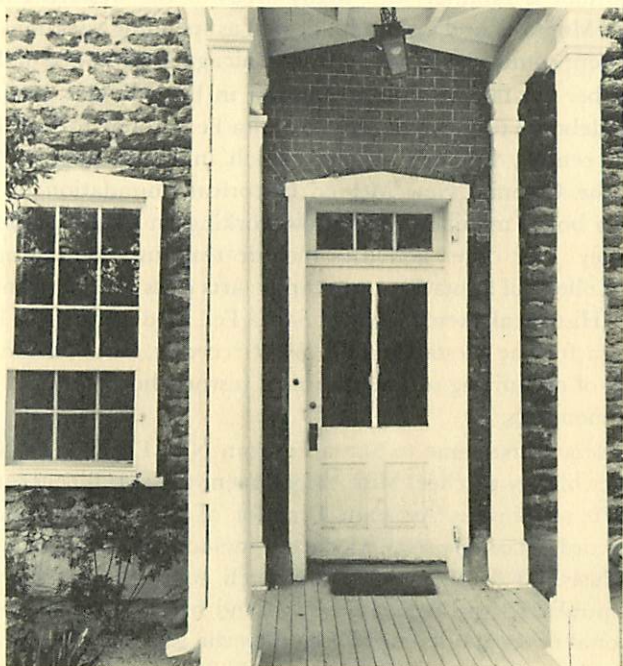
Simulated brick wall finish which was discovered under south side porch. Hope Curtis
