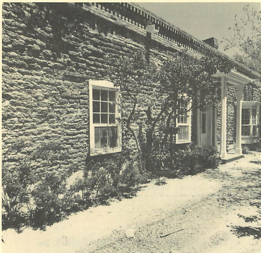
South side of the Tully House showing exposed adobe. Hope Curtis
