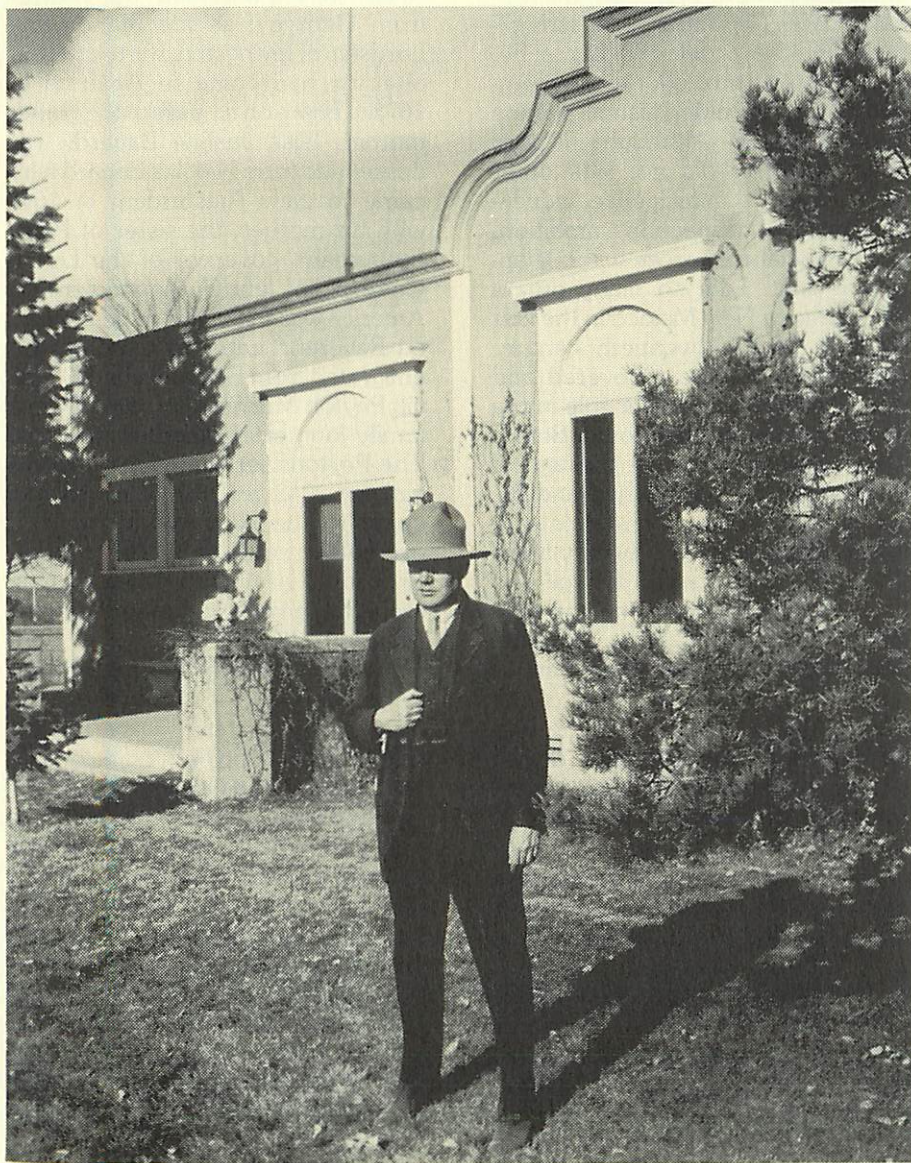
Sen. Bronson Cutting at residence Santa Fe, New Mexico
