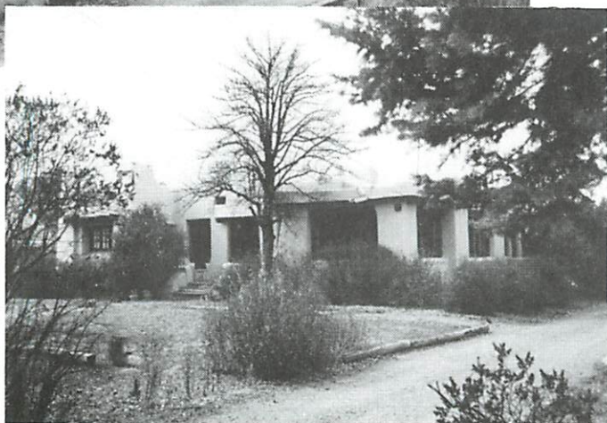
Three views of the Smith House, 1992
