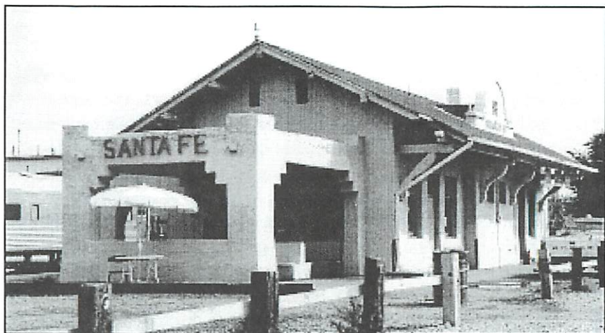
Atchison, Topeka & Santa Fe Depot. Courtesy NM Office of Cultural Affairs, Historic Preservation Division. Corinne P. Sze, photographer.
