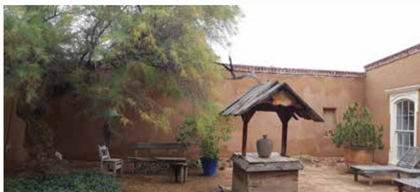
Image page 3, Garcia House west façade. Above, east façade from Vigil House courtyard. Below, Garcia House east façade.
