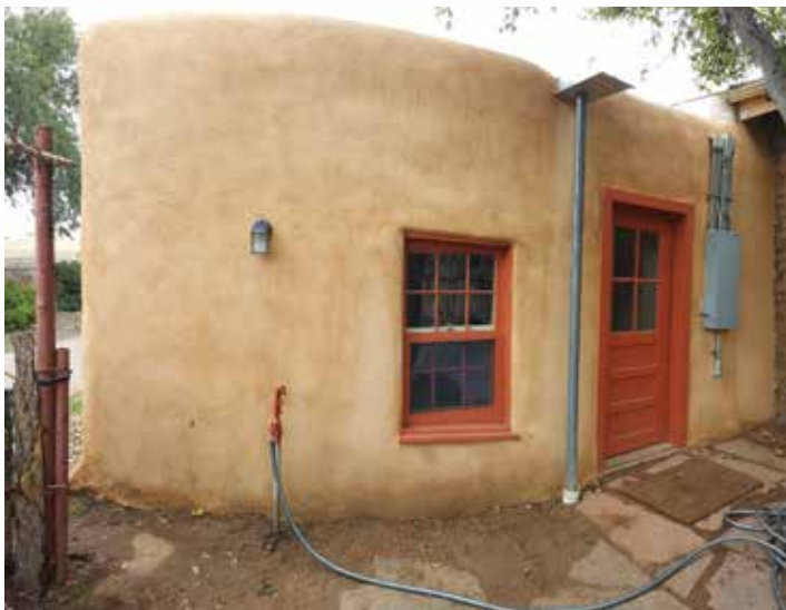
Image above Garcia House south façade.
