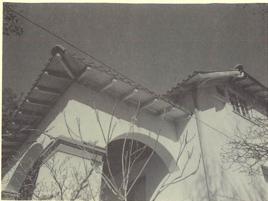
Deep hip roof sheathed in tile and by wide dormers.
