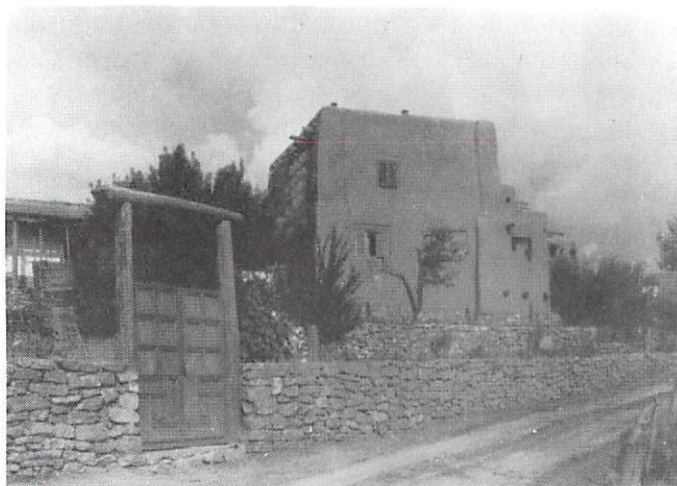
Front gate and two-story addition, Undated photo by Sheldon Parsons. Courtesy Leonora Curtin Paloheimo.
