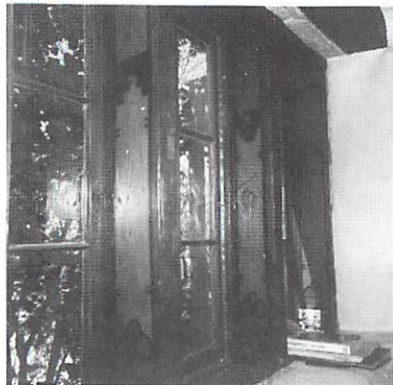
Detail on Dining Room windows
