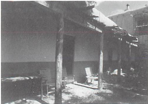
View of Portal
