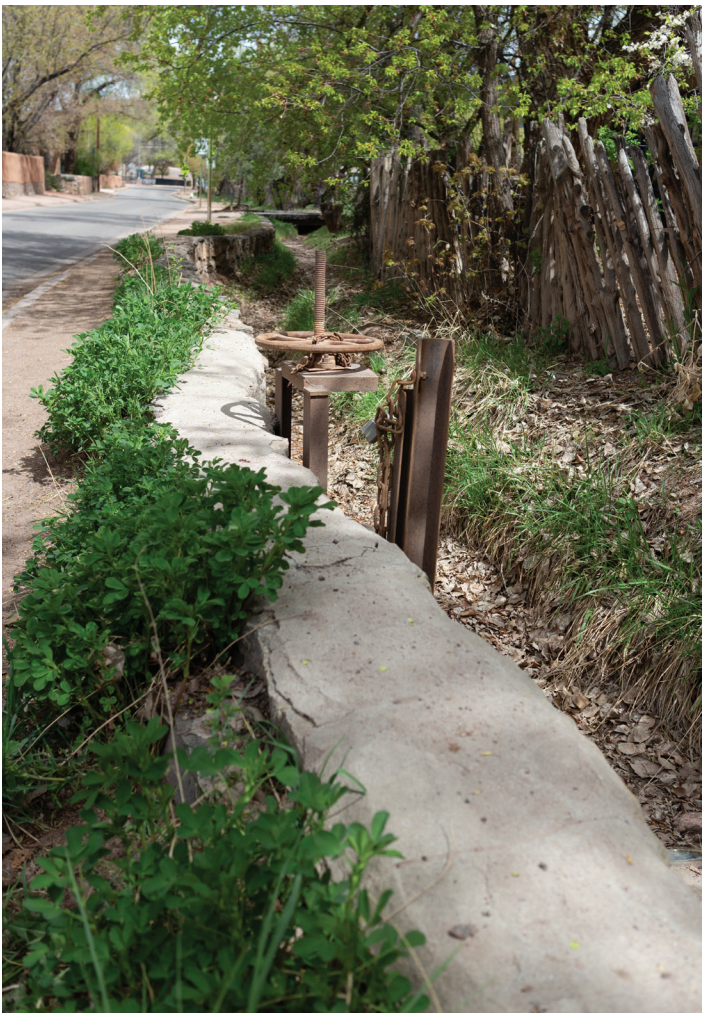
Headgate from Acequia Madre as an example of a similar device that will be installed at El Zaguán for an example of a functioning acequia. Photo by Simone Frances.
